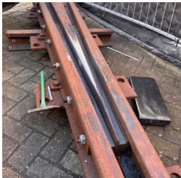
Figure 1. Rail crossing example where maintenance work will be performed. Image courtesy of RET.
